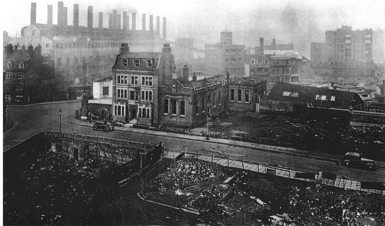
Photo. N o 3 { Existing Power Station & War-Damaged Property
